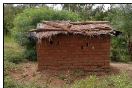
Photo 4-6 Traditional latrine (pit latrine) in the village of Kagona Mwake
